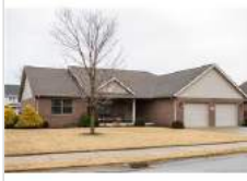
The brick façade is highlighted by neutral trim accents
